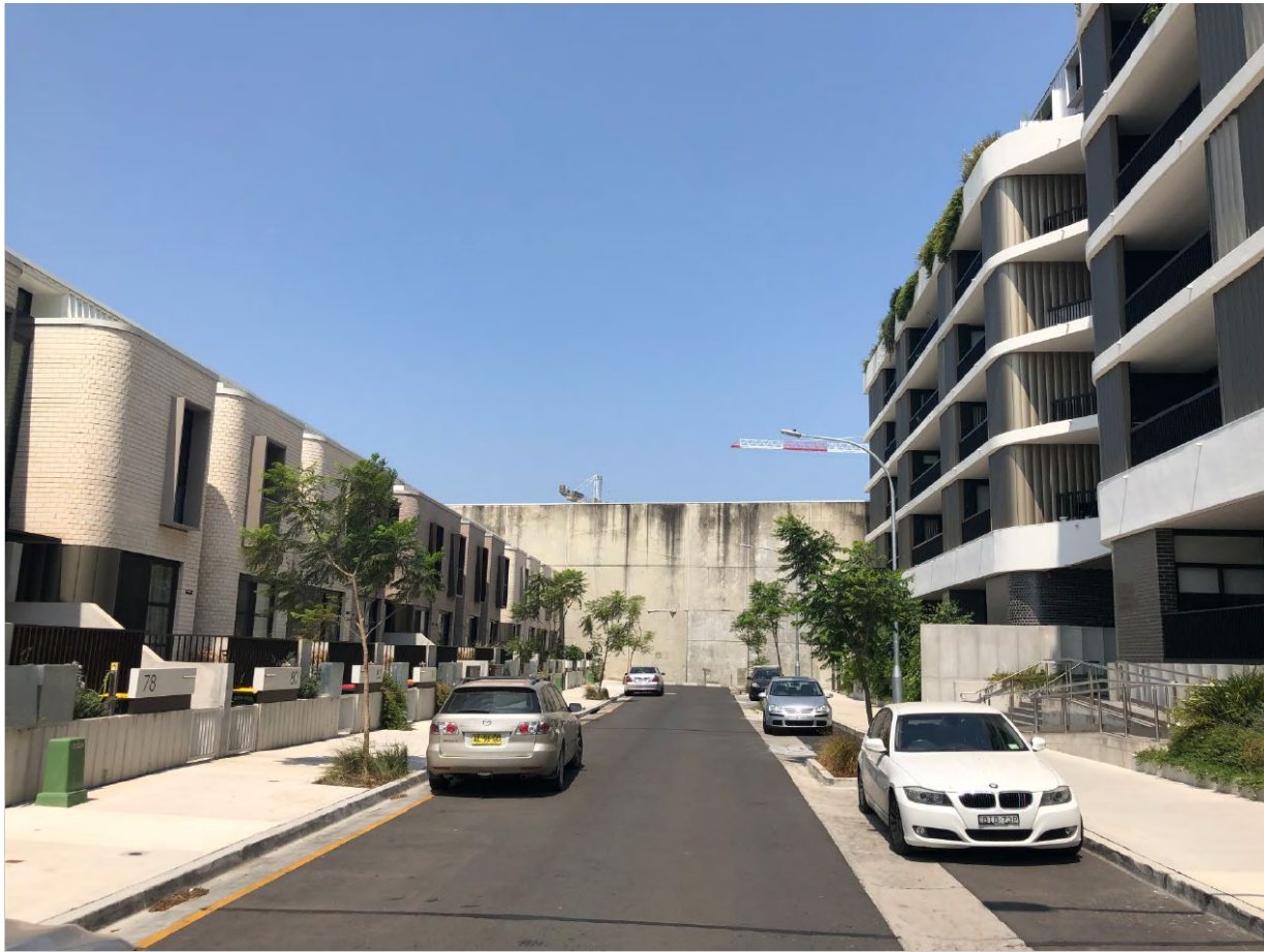
Metters Street looking east
